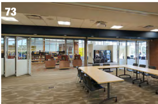
73 Nano wall to open meeting room to the lobby for overflow space for larger program attendance
